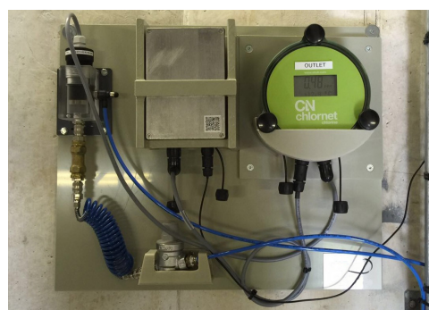
ChlorNet typical application for reservoir residual chlorine monitoring at the outlet
