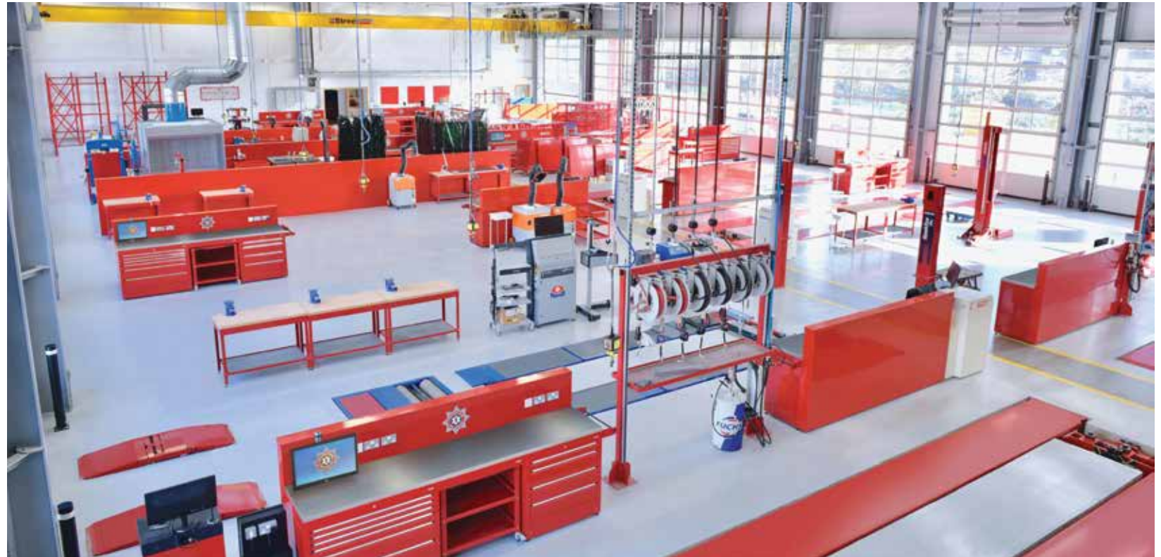
Overview of Northern Ireland Fire and Rescue Service Logistics Support Centre.
