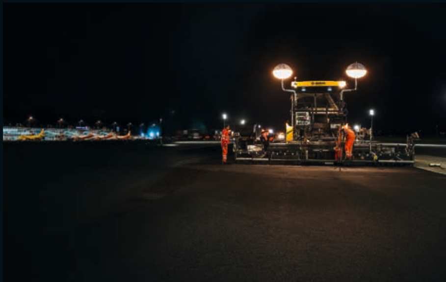
Night construction site at the airport: best laying results under time pressure.
