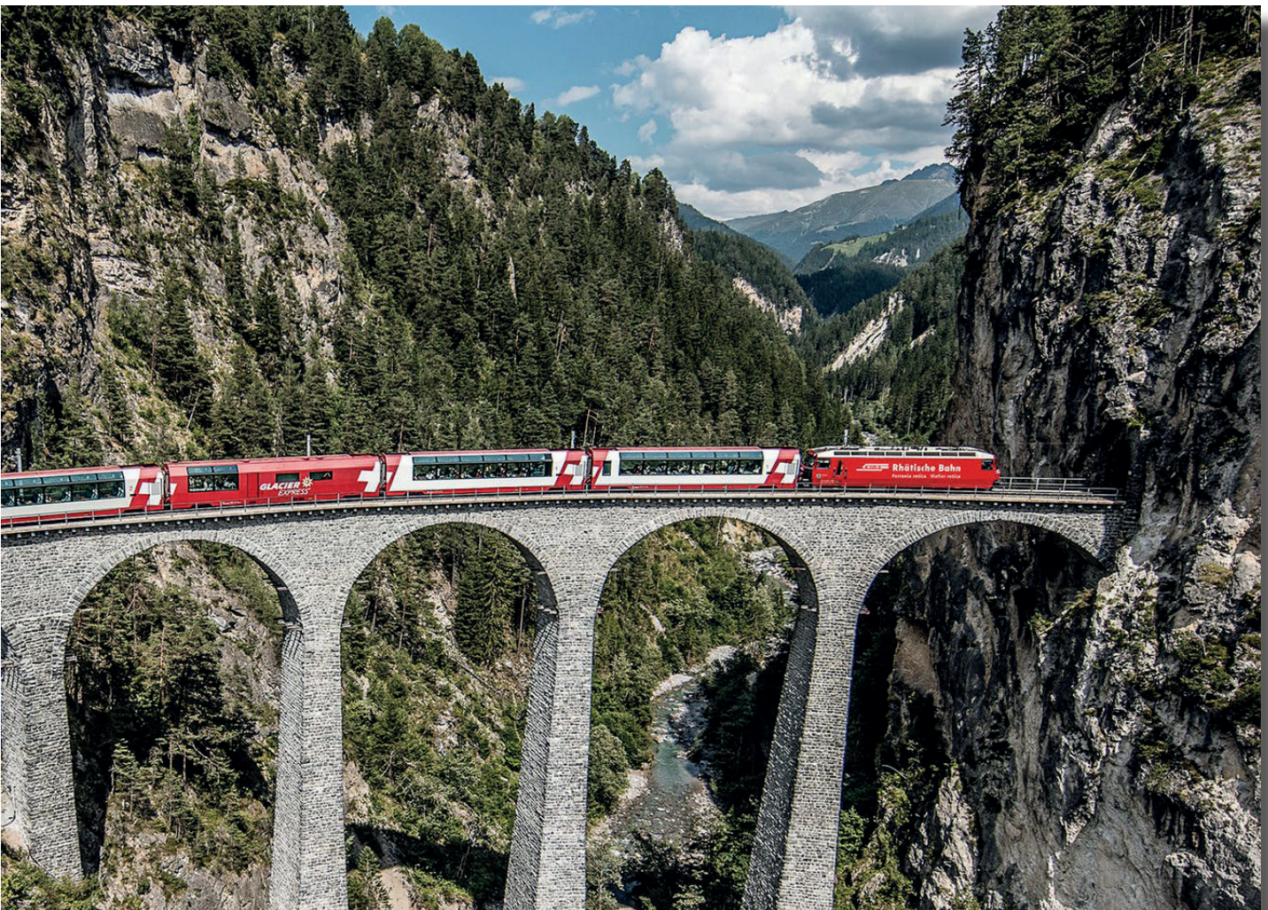
Excellence Class, Rhaetian Railways Landwasser Viaduct, Switzerland
