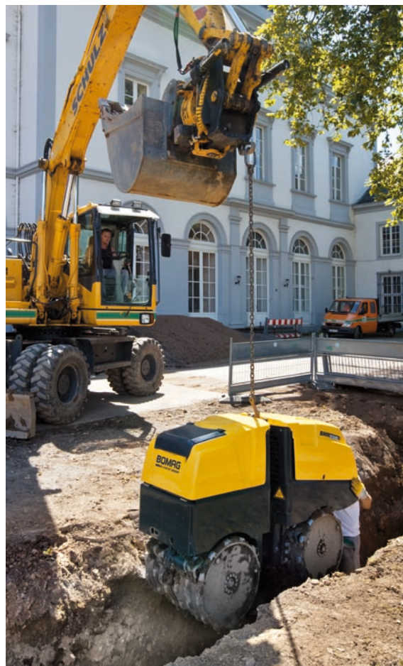
Safe and easy to transport with stable single-point lifting.
